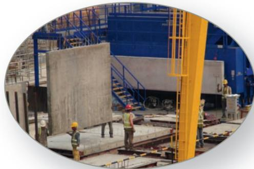
Lifting of the precast concrete elements
