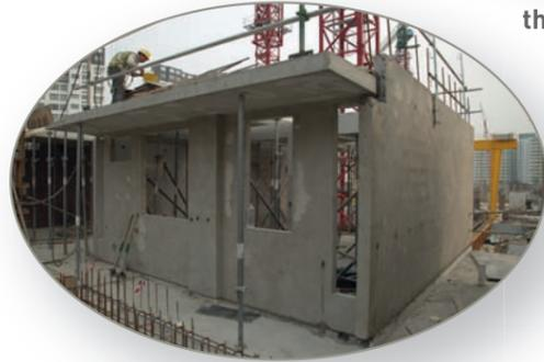
Completely installed precast concrete walls
